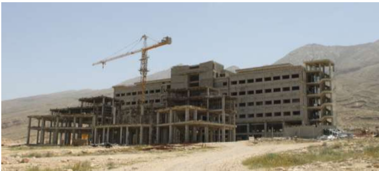
A View of the New Hospital under Construction
